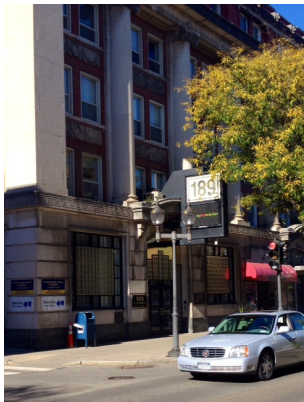
Corner of Main & Dietz Street
